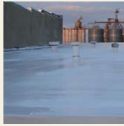
2. Prime surface with Tack Coat.
