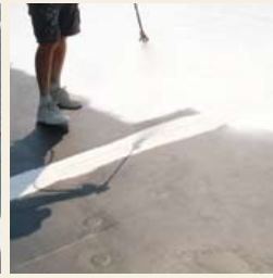
4. Seal entire roof with Rapid Roof® III Top Coat.
