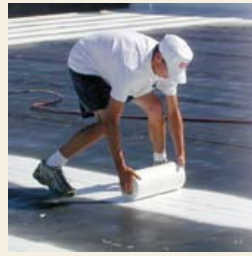
3. Reinforce seams with Spunflex® imbedded in Rapid Roof® III Base Coat.
