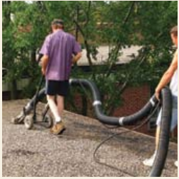
1. Prepare roof surface by removing all loose gravel and debris.
