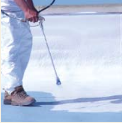
3. Coat foam surface with appropriate Conklin coating system.
