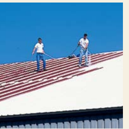
5. Seal entire roof with one of our approved acrylic coatings.
