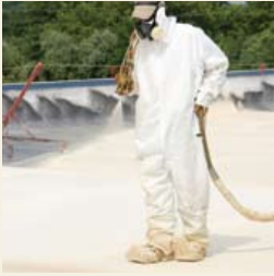
2. Apply SPF with a minimum thickness of one inch.
