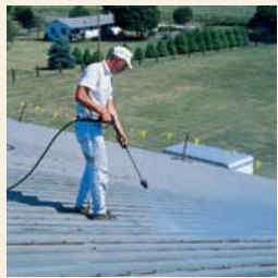
1. Power wash and clean with Rust Off® Rust Remover.
