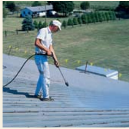
1. Power wash and clean with Rust Off®.
