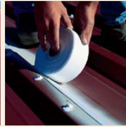
4. Reinforce existing seams with Spunflex® and base coat.
