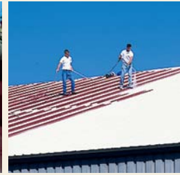
5. Seal entire roof with one of our approved acrylic coatings.
