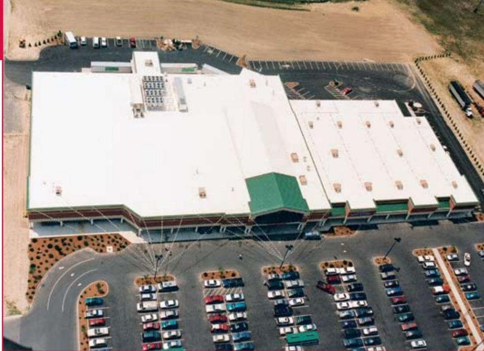
The majority of all roof jobs now use single-ply systems instead of built-up roofs. The appeal of single-ply roofing is clear, as these systems are generally more cost-efficient, longer-lasting and lighter than built-up roofs.
